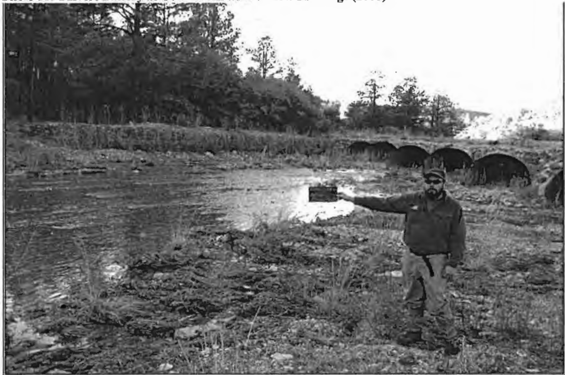
Photo 11. Culvert Battery at Coal Creek with Willow Plantings (2005)
