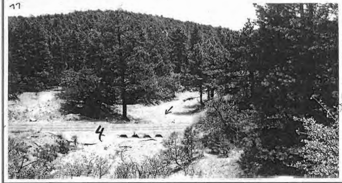
Photo 6. Original Culvert Battery at Coal Creek (1997)
