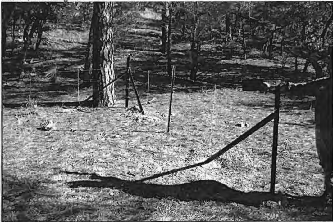
Photo 19. Fence Segment of Coal Creek Corridor
