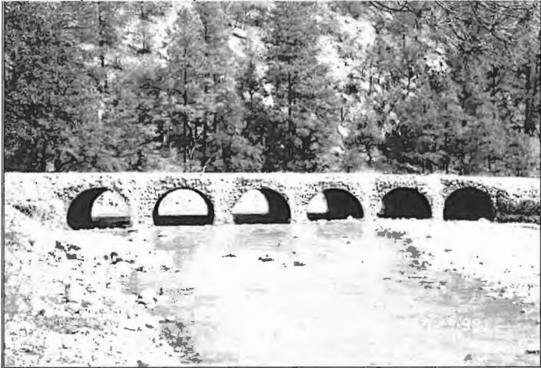
Photo 10. Completed Culvert Battery at White Mule
