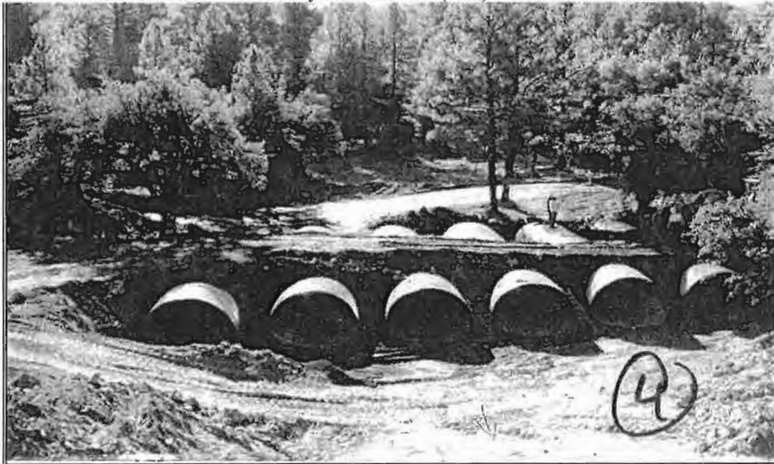
Photo 7. Construction of Culvert Battery at White Mule (1998)
