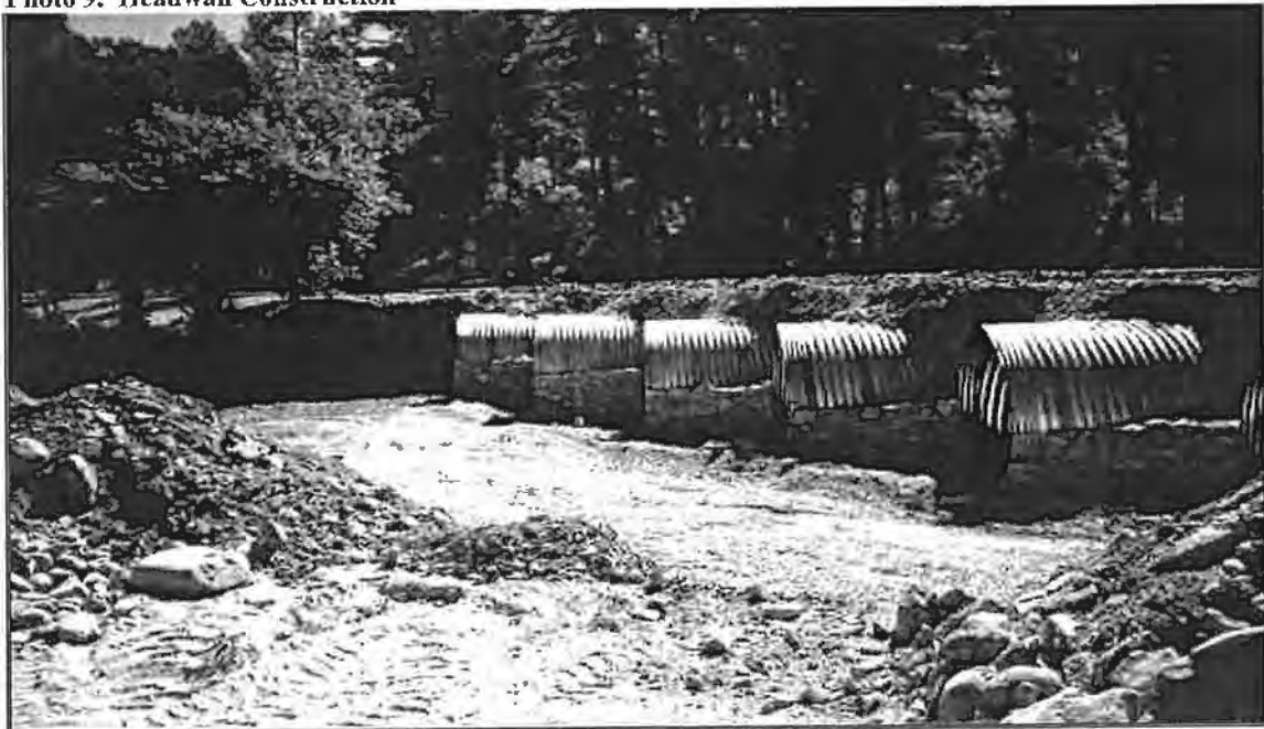
Photo 9. Headwall Construction
