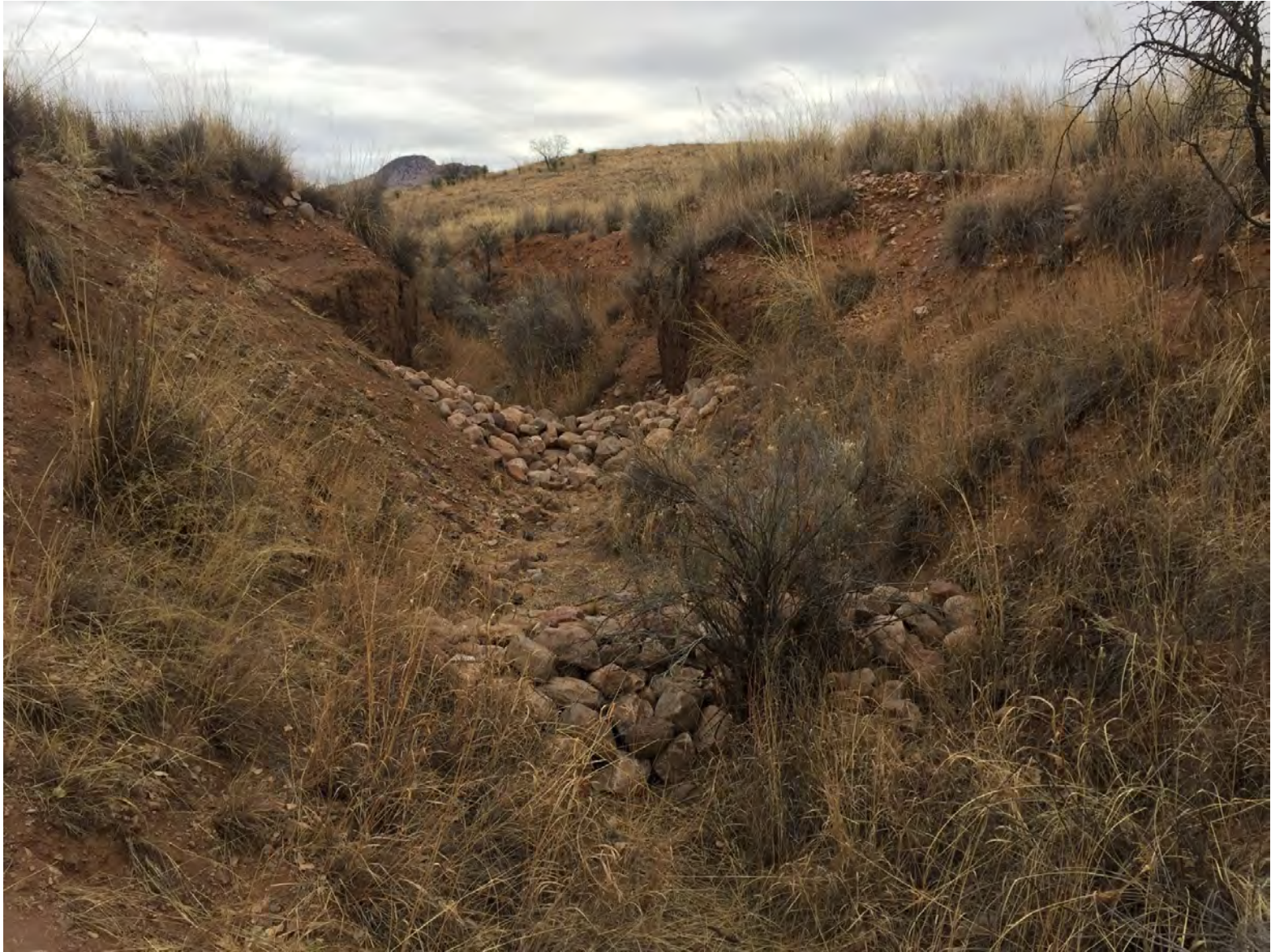
Loose rock check dams (trincheras) in the gully below Pacheco Spring
