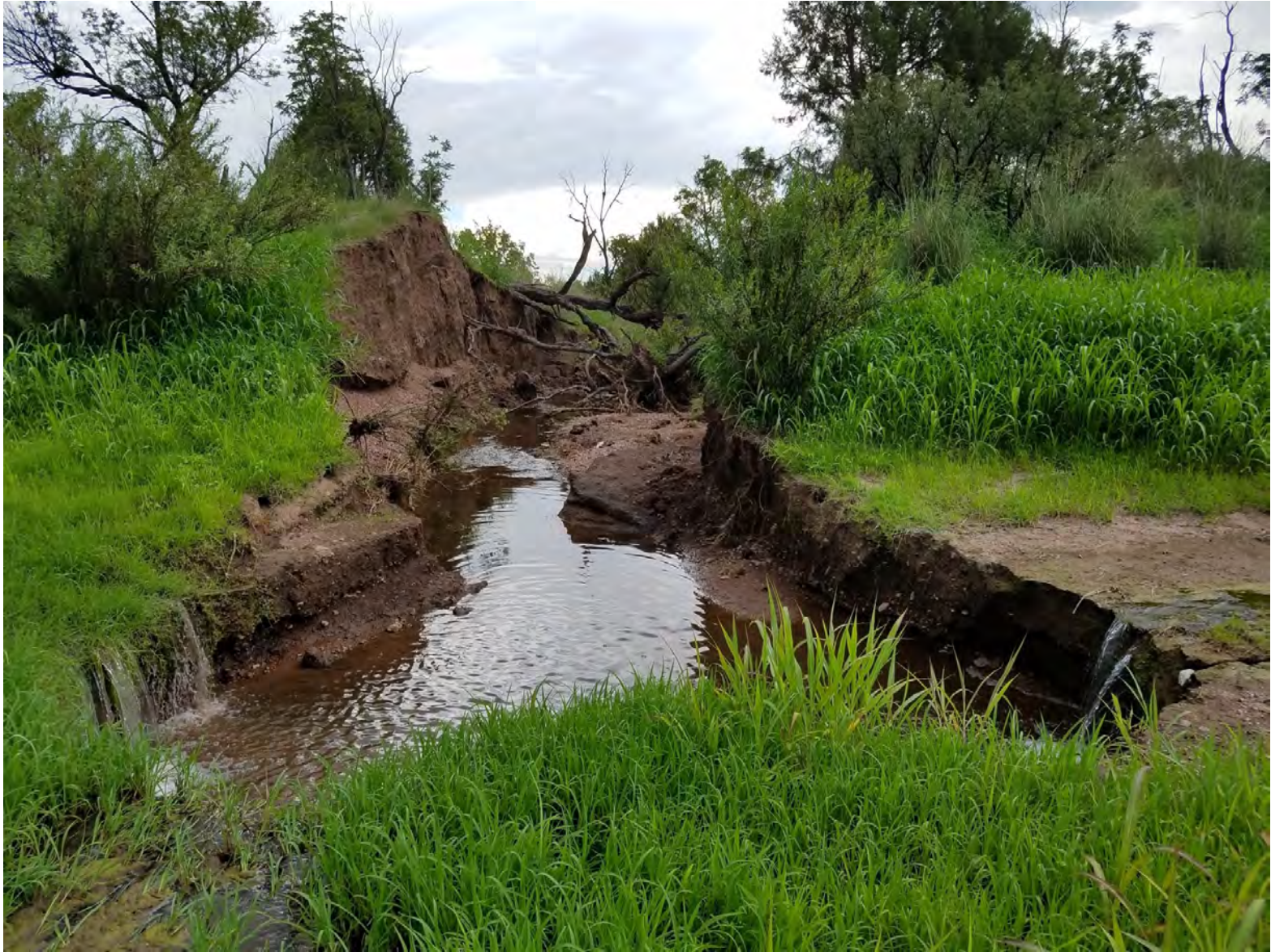
Levee cut on Diamond C Ranch-O'Donnell Canyon Ciénega after large storm event
