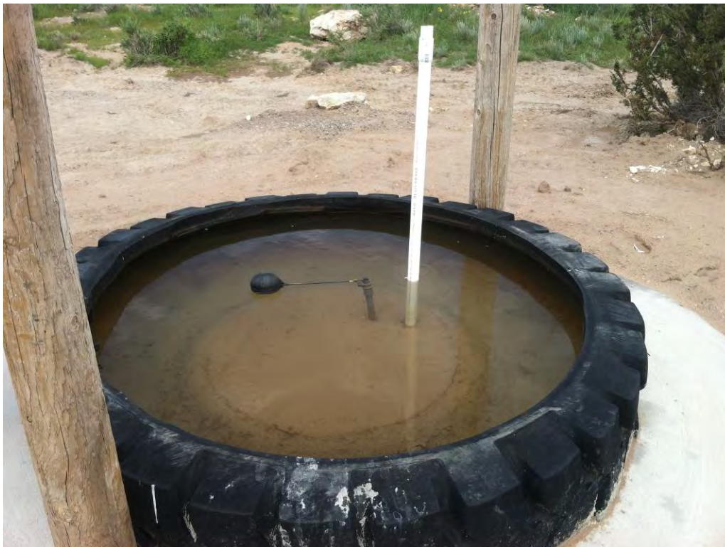
Figure 15. Newly constructed watering facility at the end of the new 8,500 ft pipeline.
