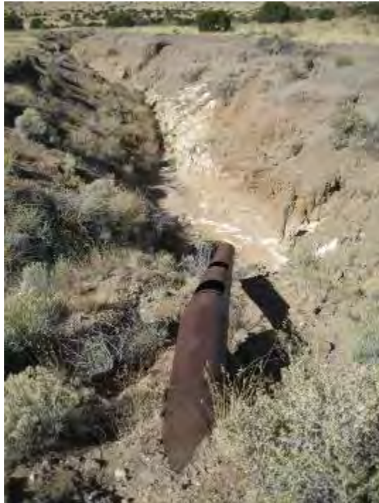
Downstream view of a detention basin; the outlet pipe is undersized and causing severe erosion.
