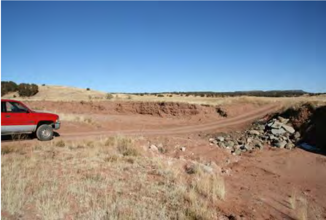
A failing grade-control structure at a road crossing on a tributary to Coyote Creek.
