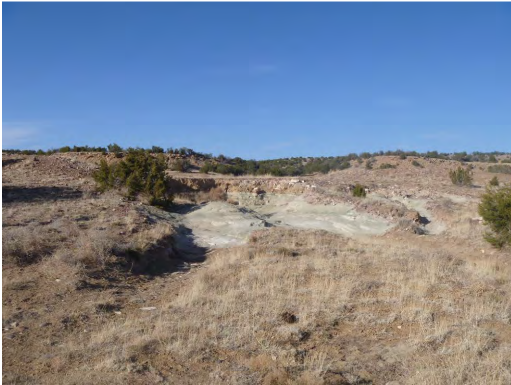
Figure 11. Eroding sediment basin spillway.
