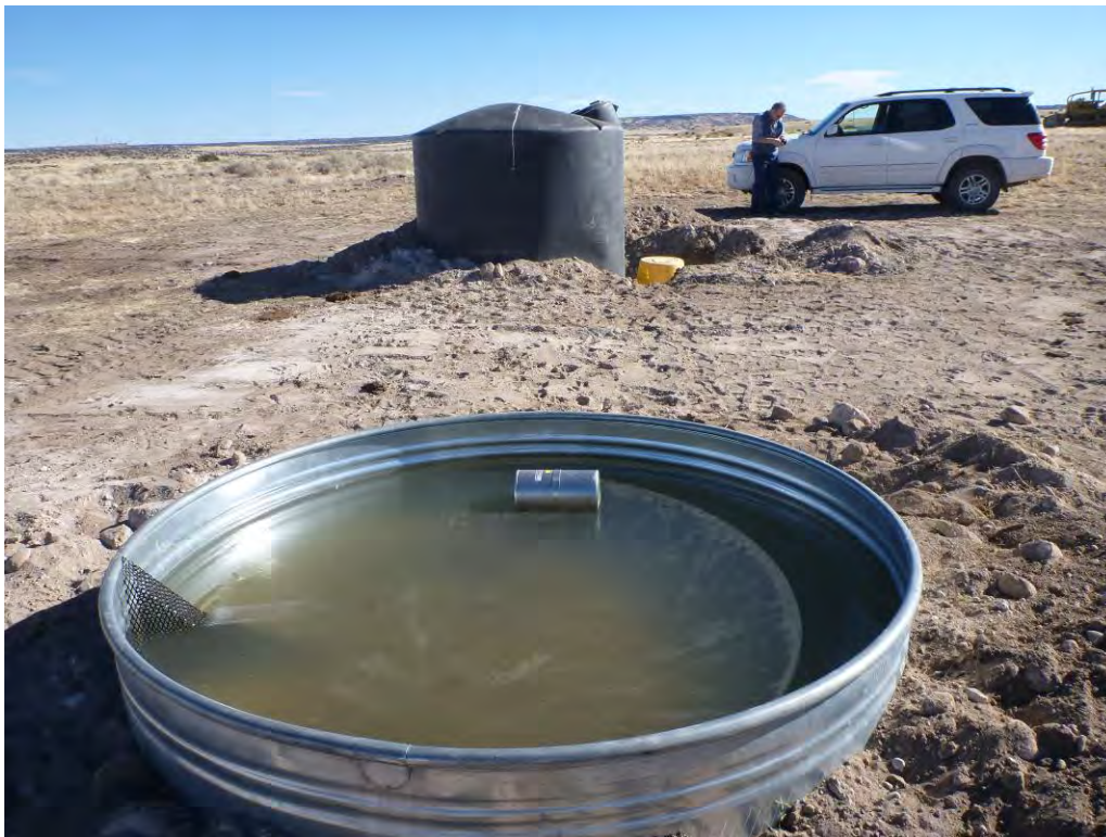
Figure 7. Trough and storage tank at the end of the pipeline.
