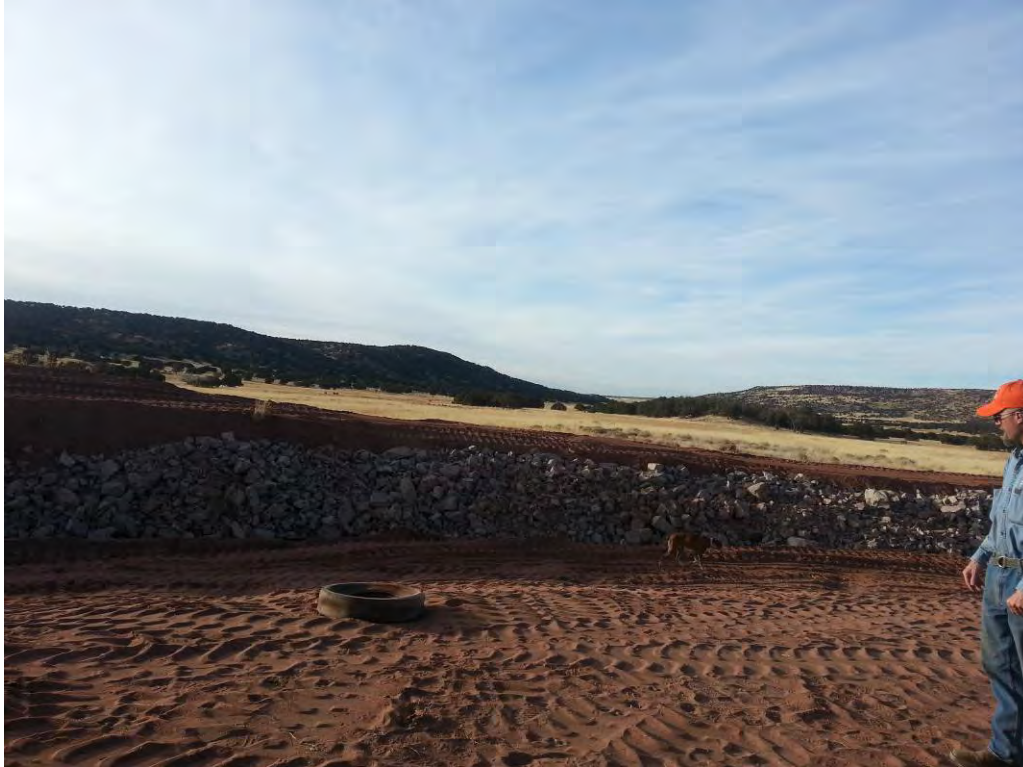
Figure 9. Post construction photograph of the repaired berm with rock protection.
