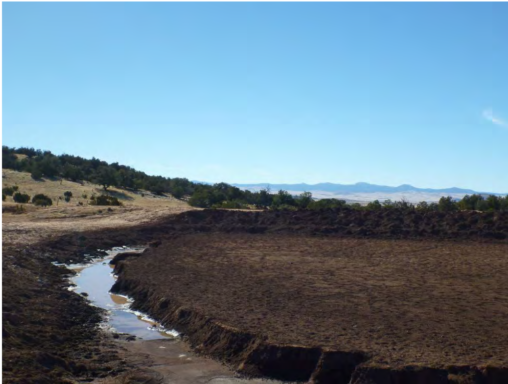
Figure 4. Excavation of sediment from the stock pond.
