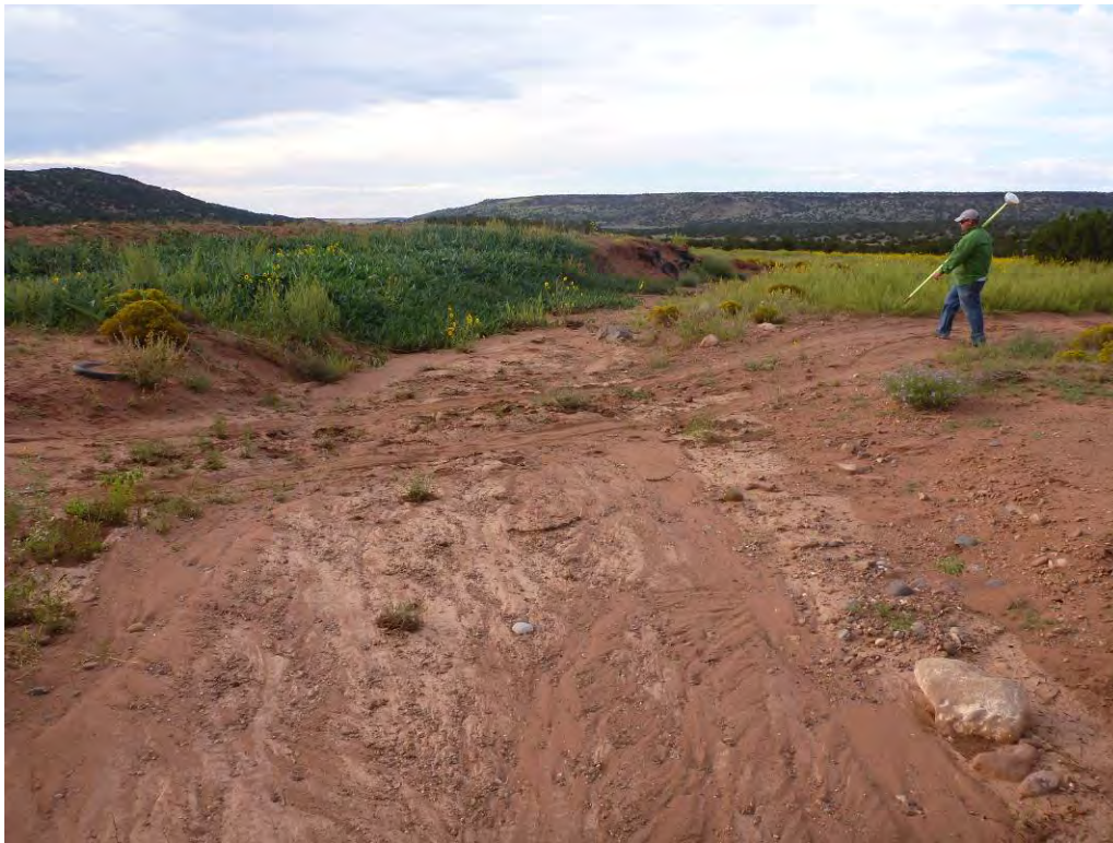
Figure 8. Surveying the failed berm prior to construction.
