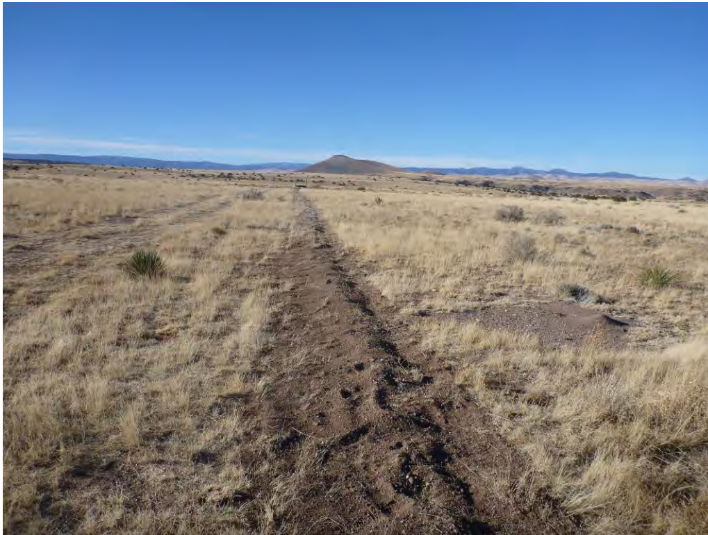
Figure 13. Buried pipeline with spoil mounded above trench.
