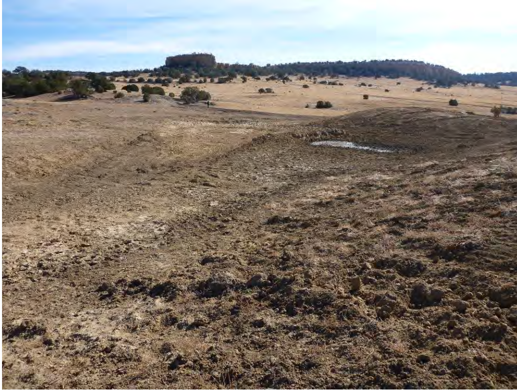
Figure 12. Post construction photograph of the sediment basin with linear spillway.
