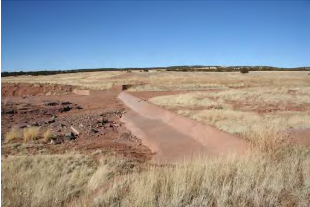
Grade-control sill has effectively controlled the course of Coyote Creek and maintained the local grade.
