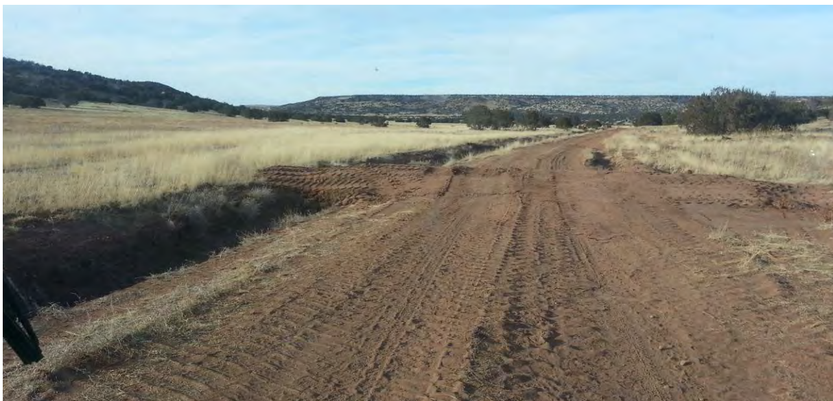
Figure 10. Construction of a roadway drain dip.
