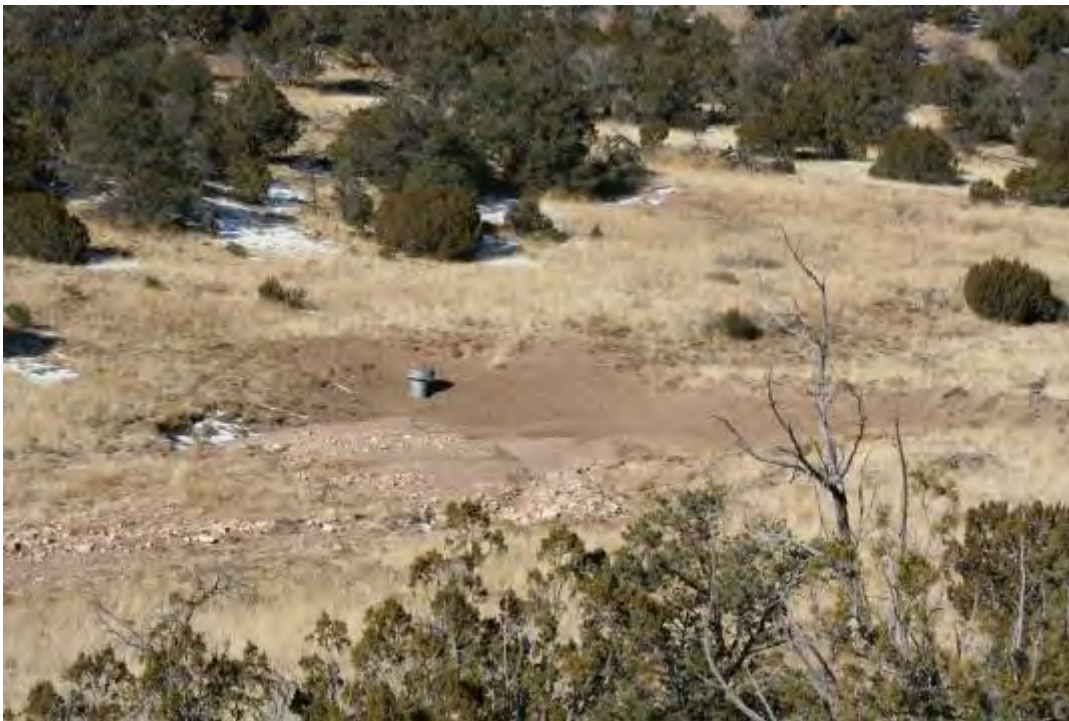
Shows a failed WASCOB that has reached the end of its service life and is potentially built in a location that has too large of a contributing watershed.
