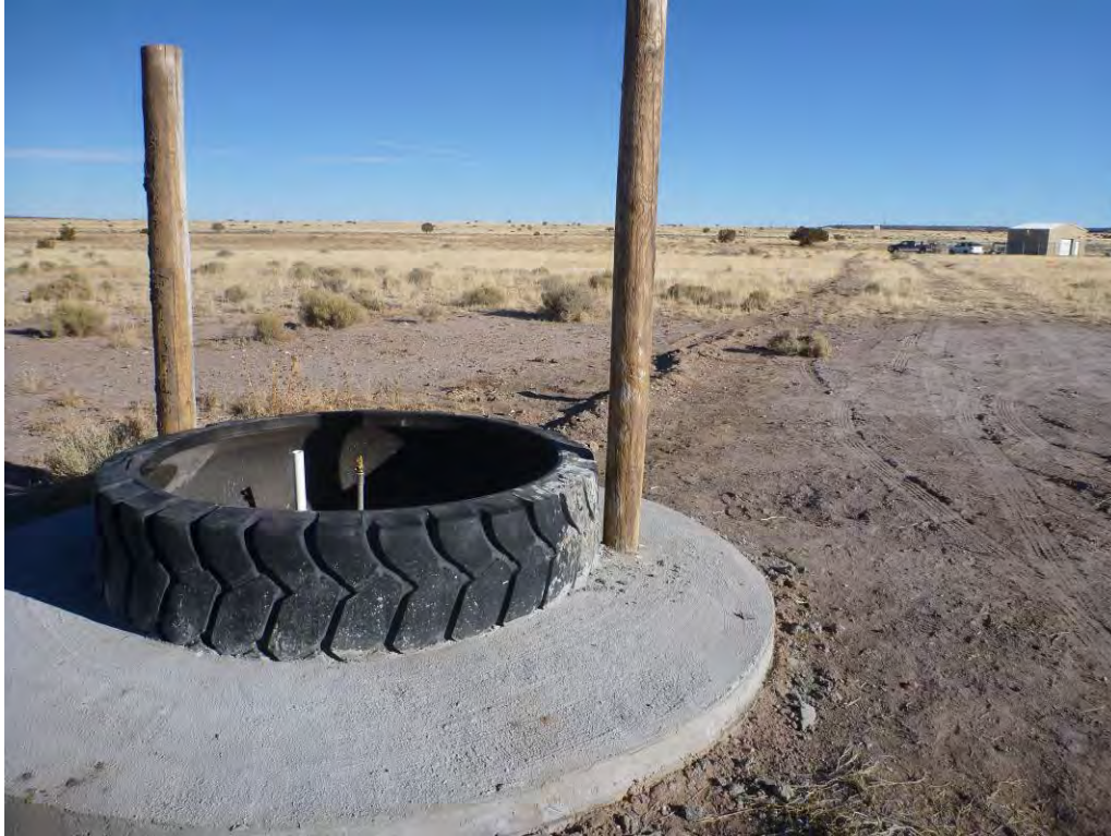
Figure 14. Newly constructed watering facility at the end of the new 450 ft pipeling.
