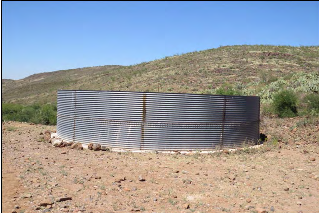
Figure 5. Storage tank looking northwest. Goat Camp Pasture – Twin C Allotment. 9/30/2015.
