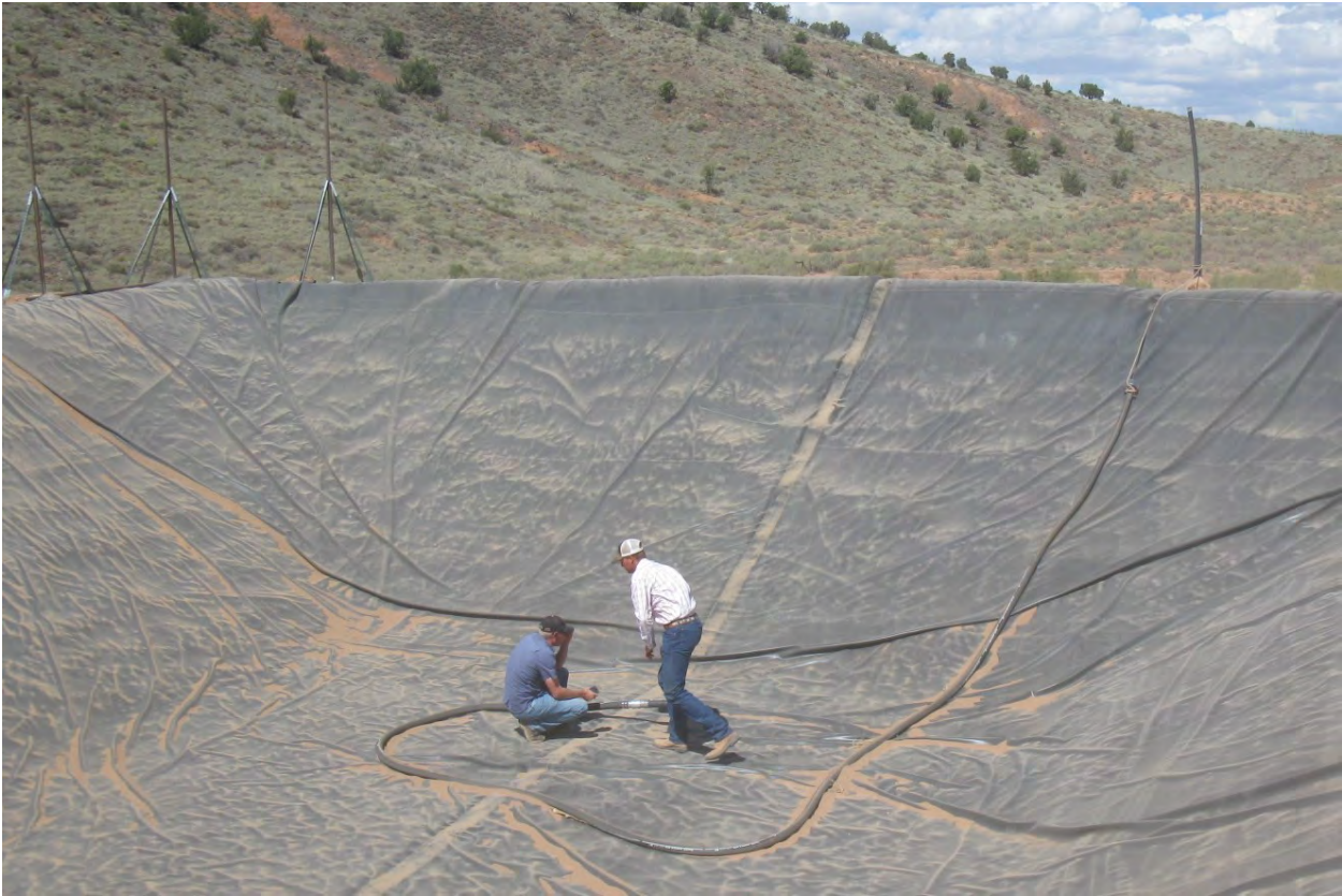
Figure B.2. Lined Storage Pond.
