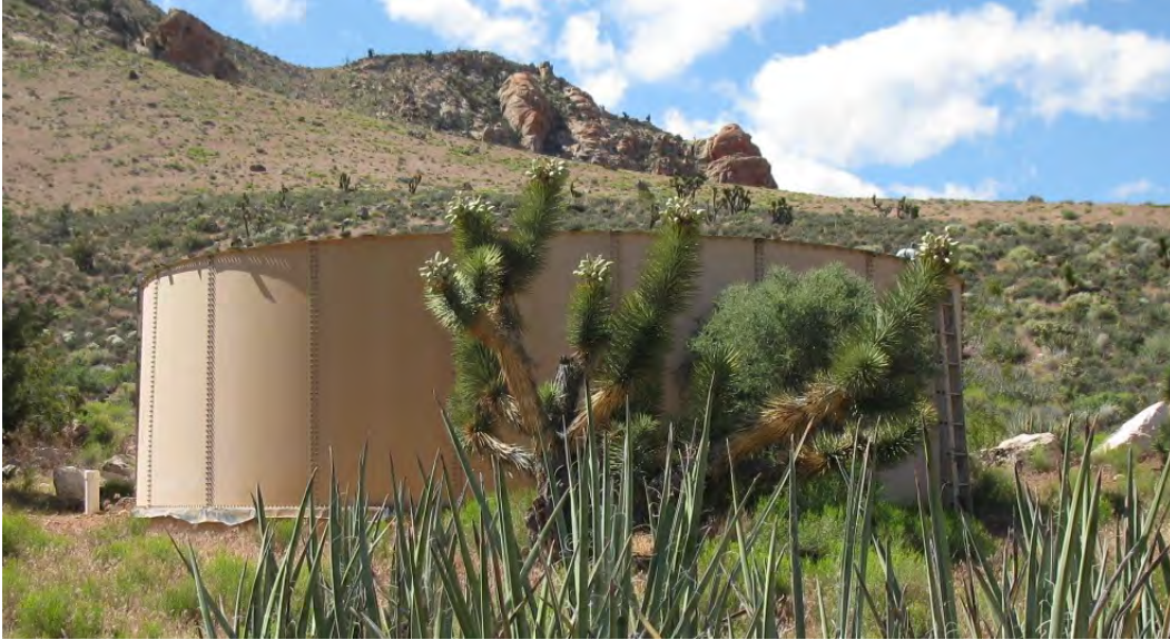
Figure B.3. Metal Storage Tanks.
