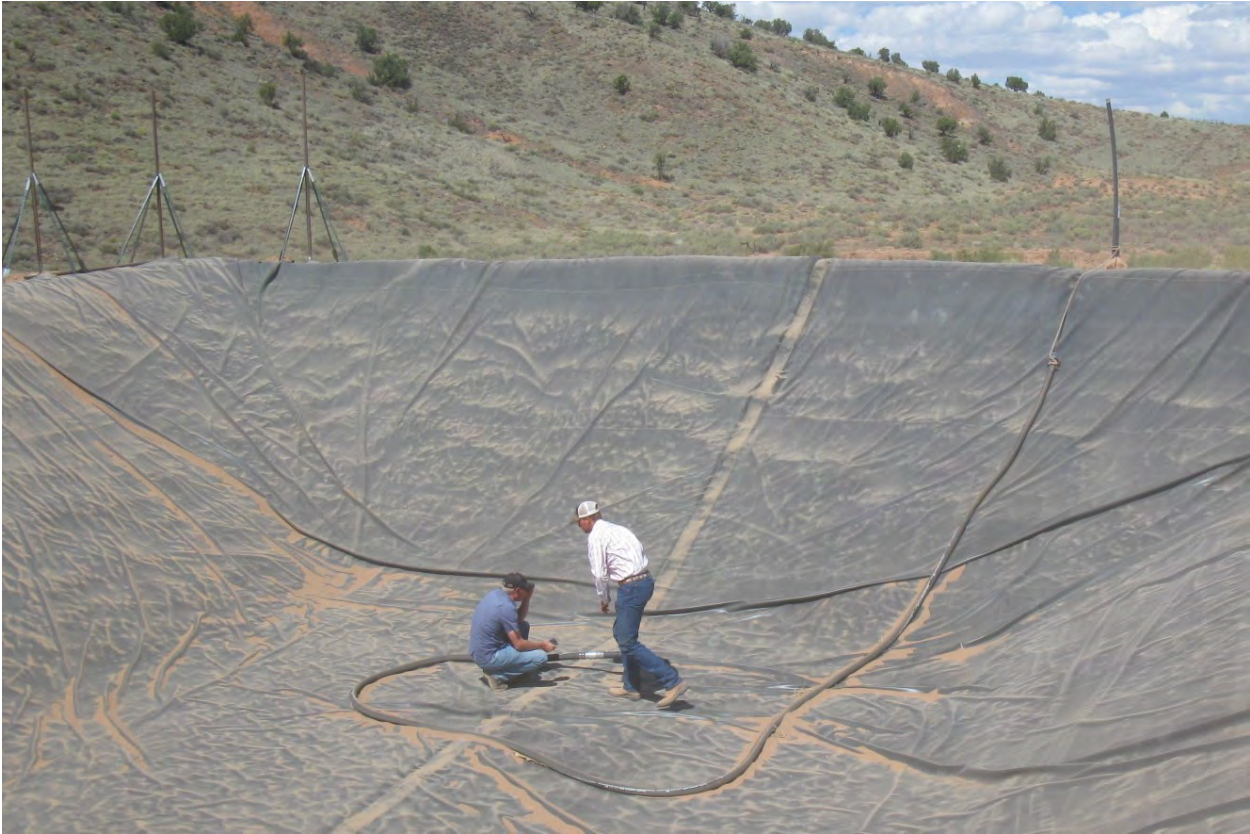
Figure B.2. Lined Storage Pond.
