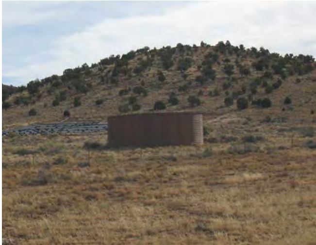
Figure 13. Water Storage Tank.
