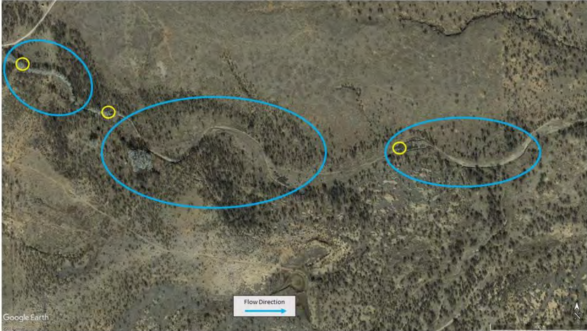
Figure C-15. Empire Gulch, downstream of BLM 6901 road; large headcuts are demarcated with yellow circles, and blue ovals indicate areas where one-rock-dams will be installed.
