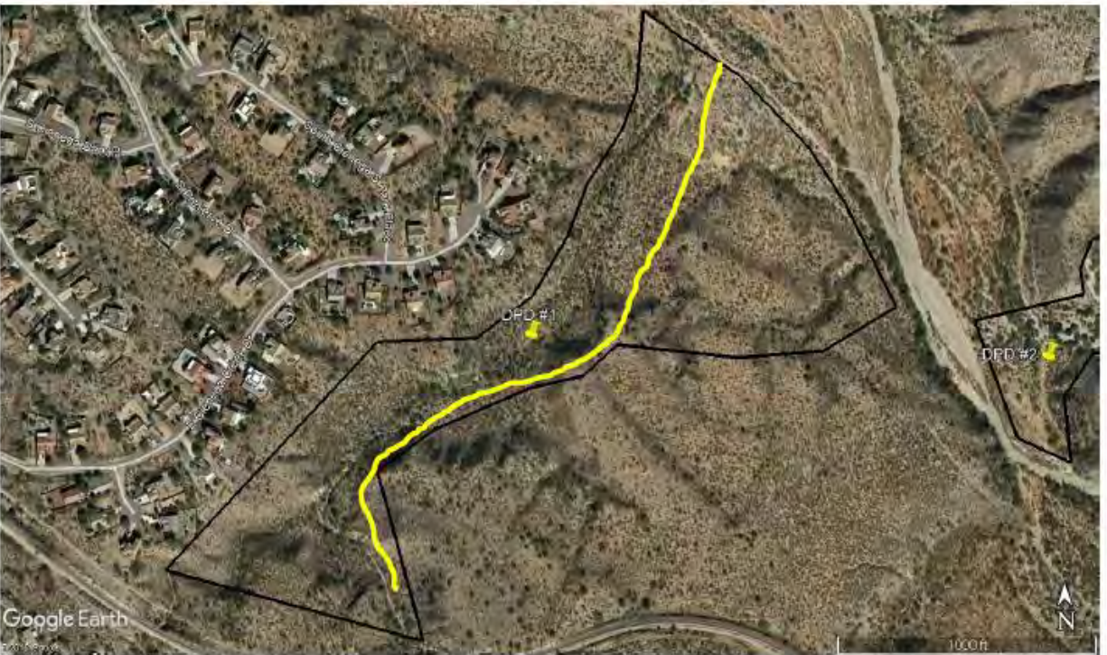
Figure C-14. Downstream Pantano Dam #1: Top photo: Access and Staging Area, Bottom: Area of potential effects in black, access road in yellow.
