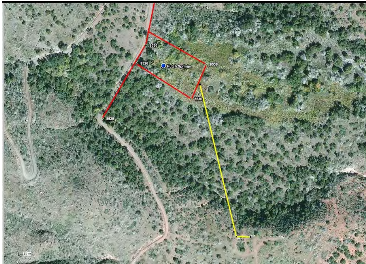
Figure 1: Aerial image of Hutch Springs with approximation of where pipe rail fencing (in red) to be installed, and water pipes (in yellow) to be installed to support the existing drinkers on the ridge to the south.
