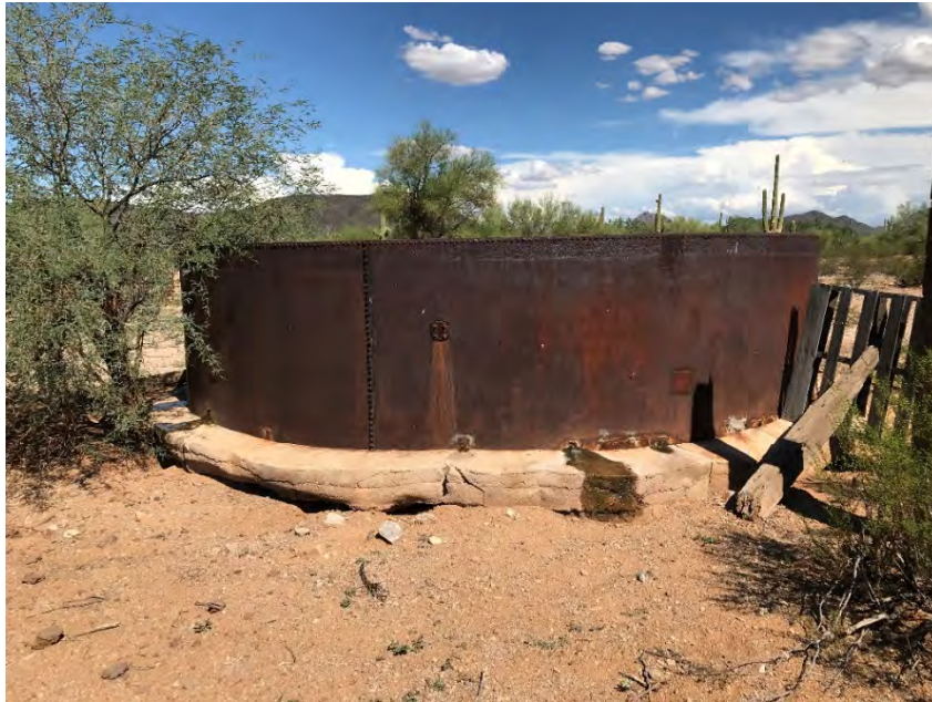
Existing Storage Tank at High Horse Corrals
