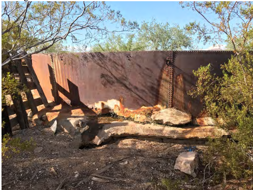
Existing Storage Tank at South Corrals
