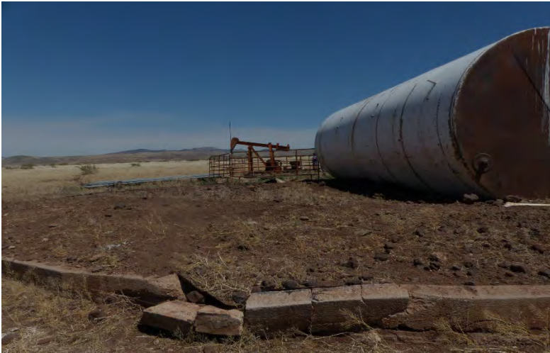
Back Pasture Well and Storage Tank
