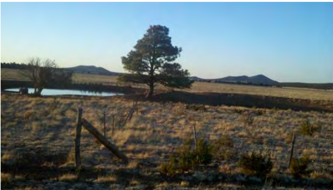
Potato Tank is actually two tanks one holding water and the other one which has failed (Pictures taken by Copper State Earth Works, 2014).
