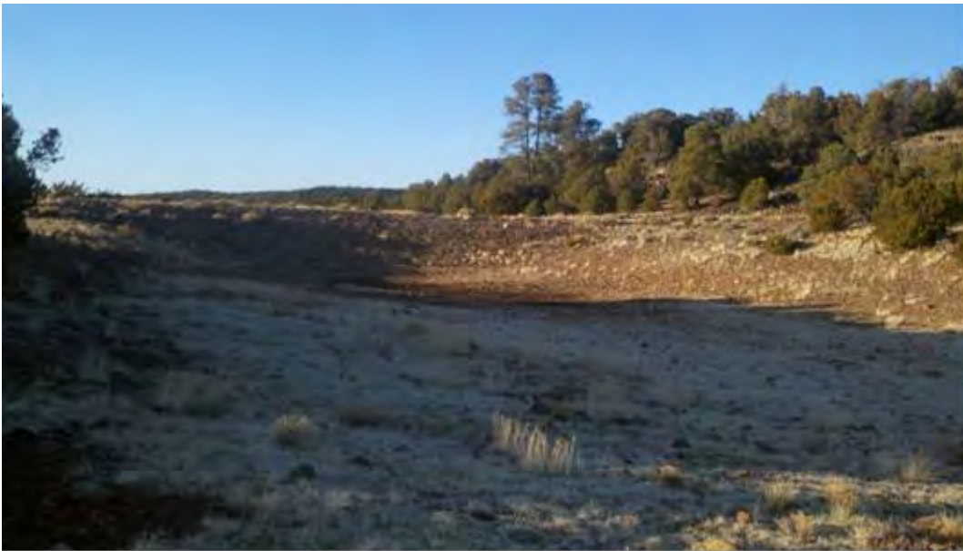
Hibbon Tank which is completely dry (Pictures taken by Copper State Earth Works, 2014).
