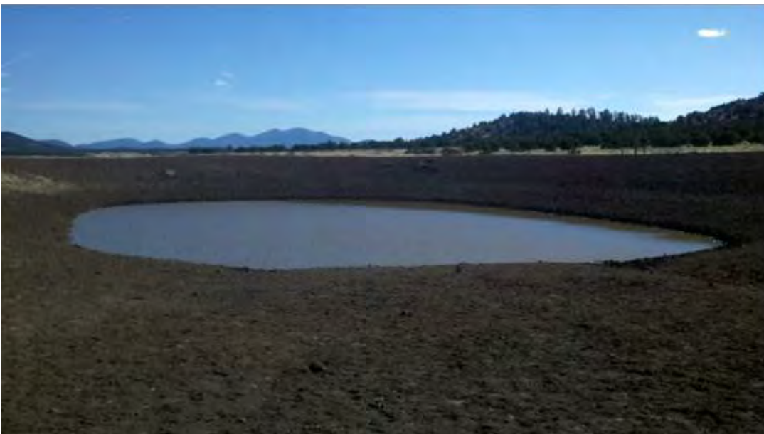
Butcher Knife Tank with approximately 4' of water (Pictures taken by Copper State Earth Works, 2014).
