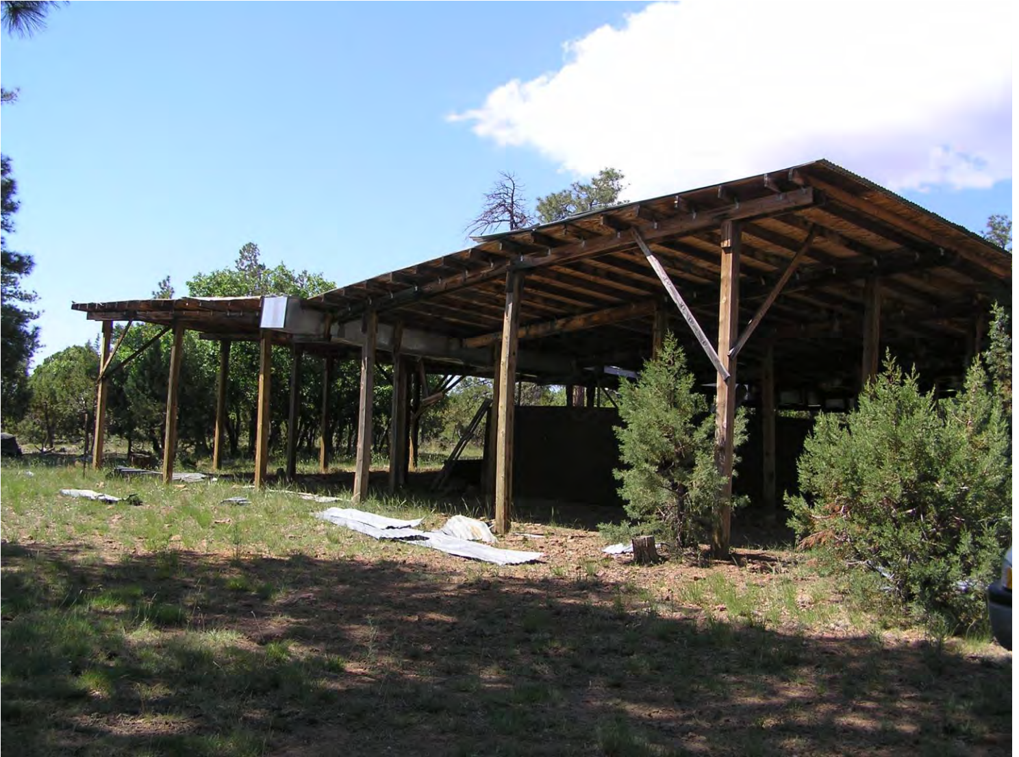
Photograph 2 Photograph of Pinetop Mountain Catchment looking southwest.
