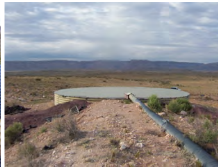
Higley Tank Lid After
