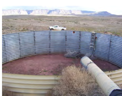
Higley Tank Before
