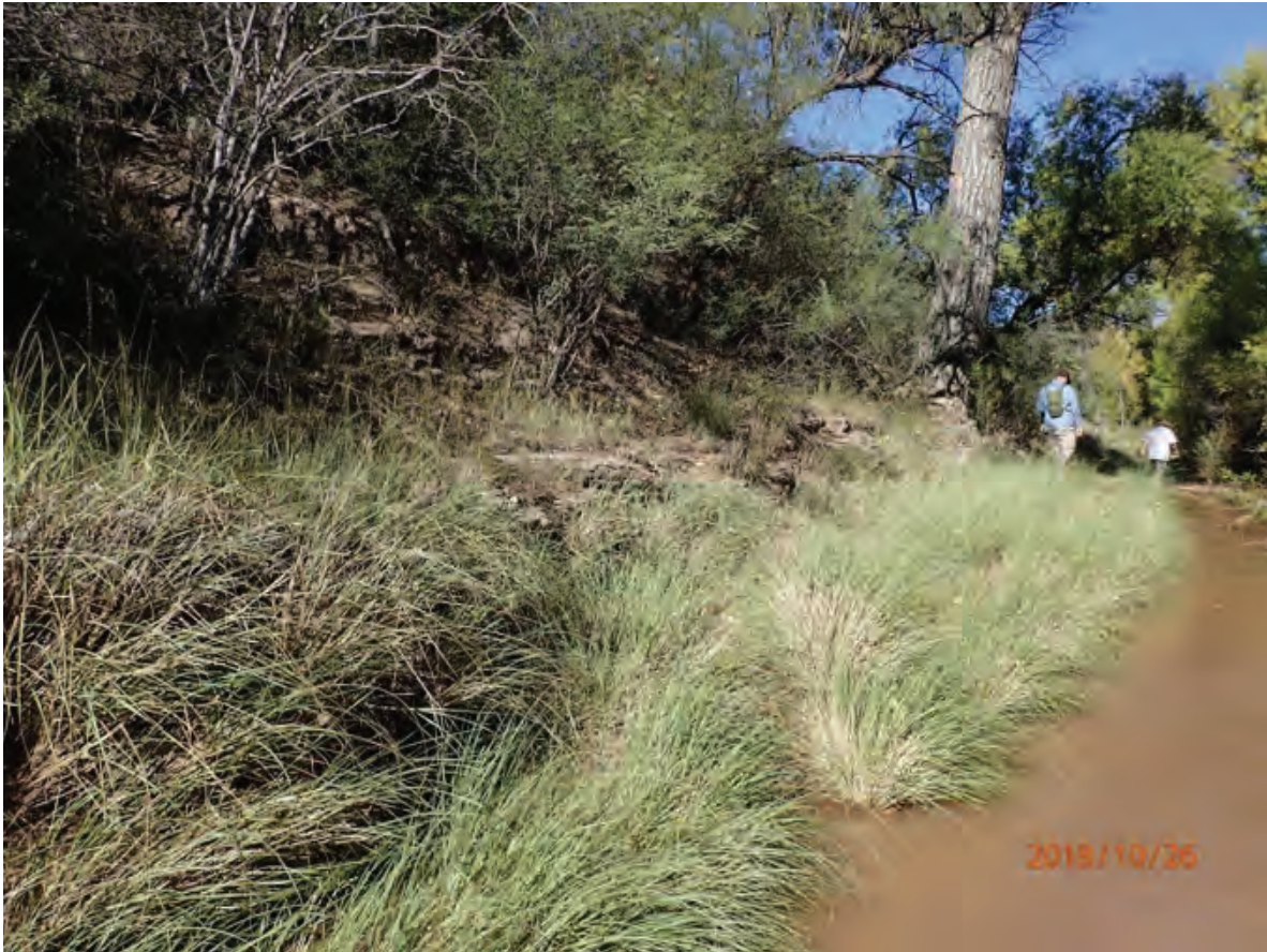
Figure 9. Stable bank in confined portion of river reach. Note large cottonwood root extends along bank above deer grass. Bank stability is excellent at this location.
