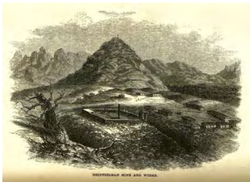
Figure 6. Bird's-eye View Drawing of the Heintzelman Mine ca. 1863 (aka. Cerro Colorado; from Browne 1871)
