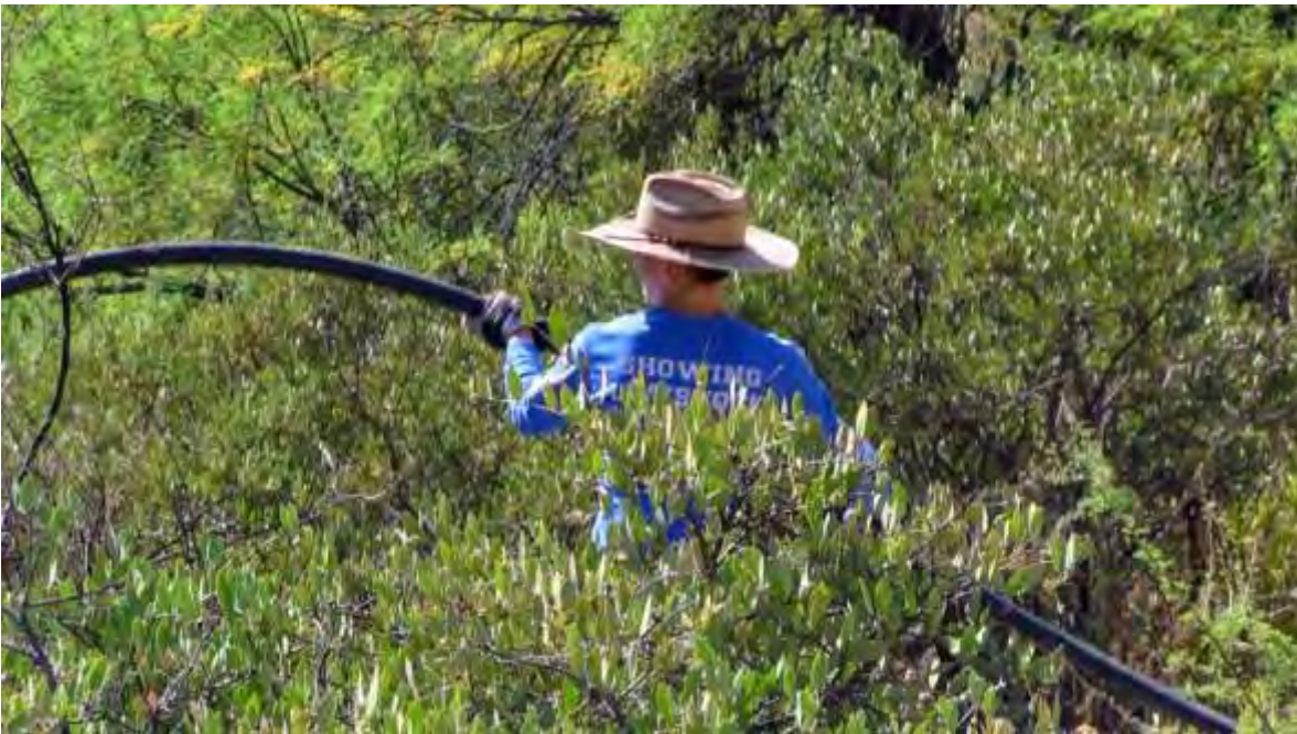
PHOTO 5; Installing Pipe for the Desert Bighorn Sheep Water Pipeline Project
