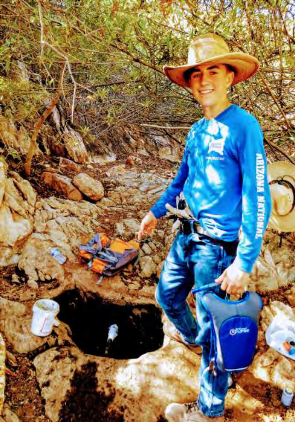
Christian Lueck, Eagle Scout Project at Completed Spring Collection Box for Desert Bighorn Sheep Water Pipeline Project
