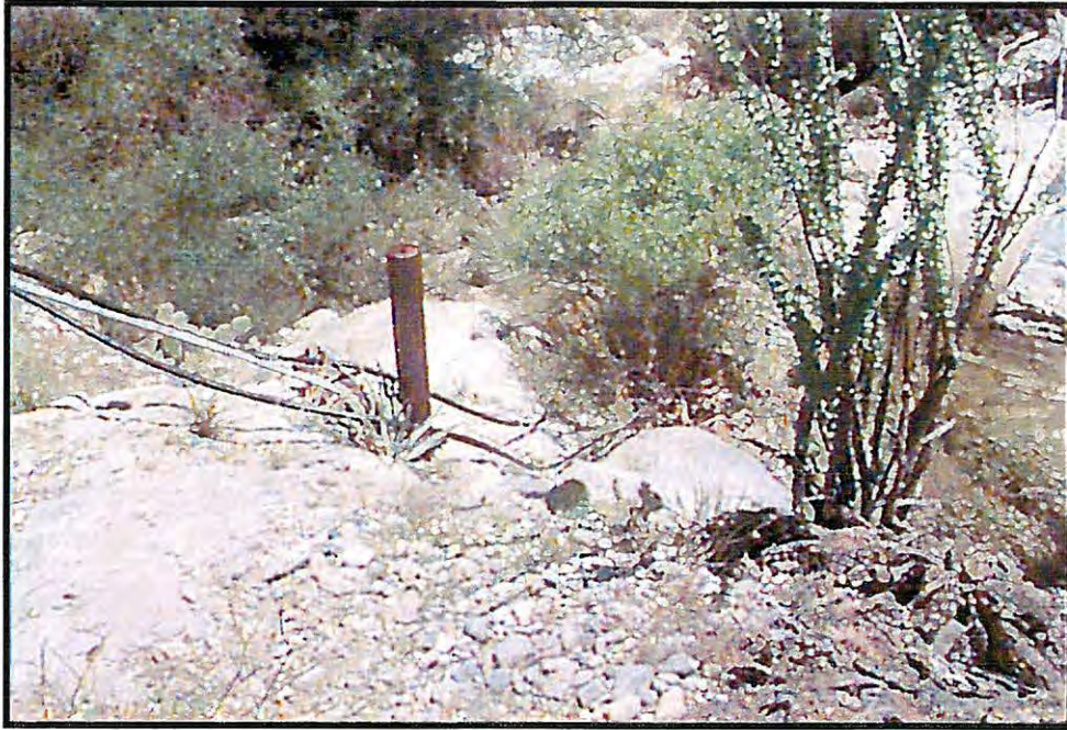
PE pipeline replacement to 5 HP pump at Youtcy Spring. N64°E.
