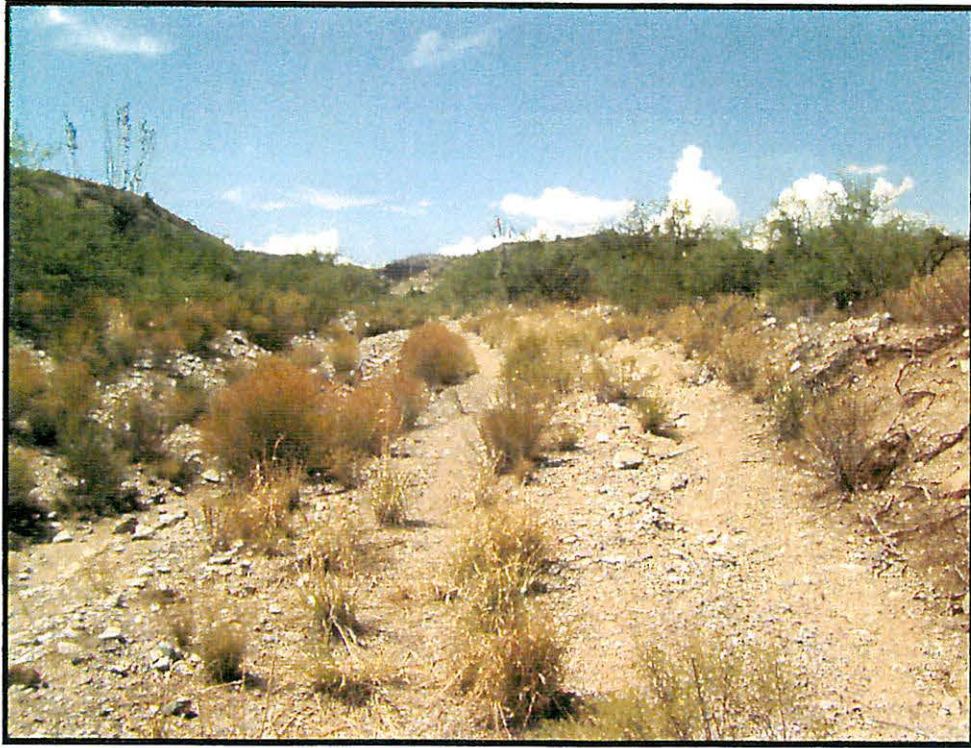
Broken water line. S175°E. Replacement required.
