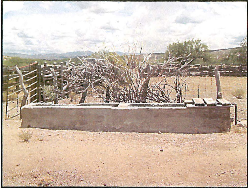
Functional White House trough #5. S110°E. No replacement required.
