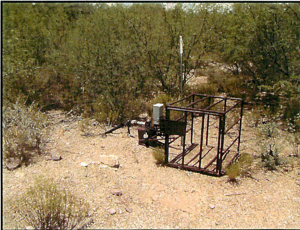
Hughes well upgrade. N286°W. Pull pump and upgrade to 1½ HP.
