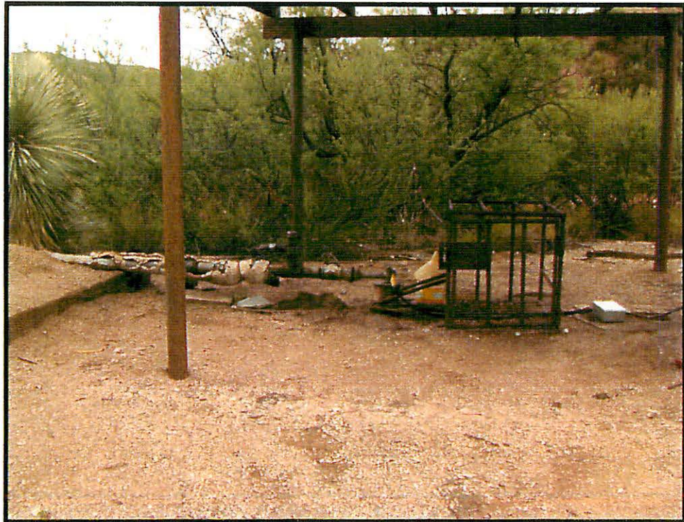
New water line to Bar LY well. S170°E
