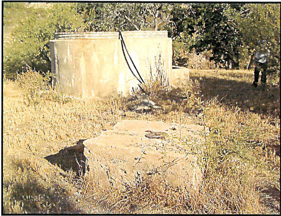
Seep Tank well N306°W. Well location for upgrade.
