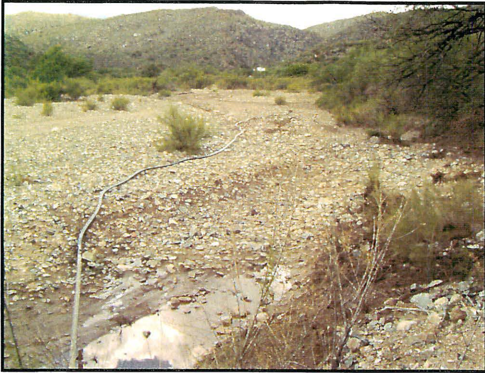
Bar LY waterline replacement. S224°W.
