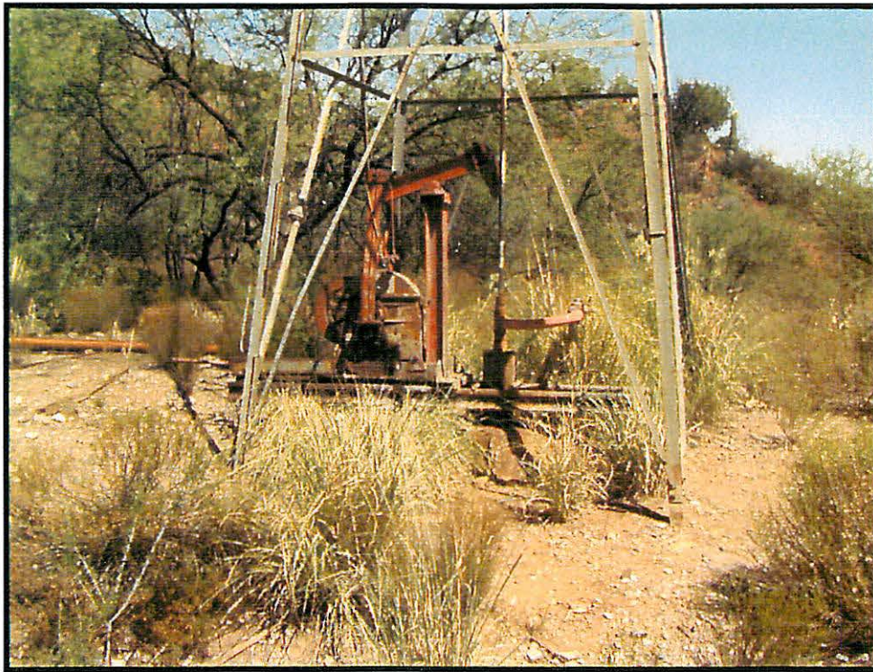
Roble West windmill. N328°W. Install submersible pump and fish out drop pipe.
