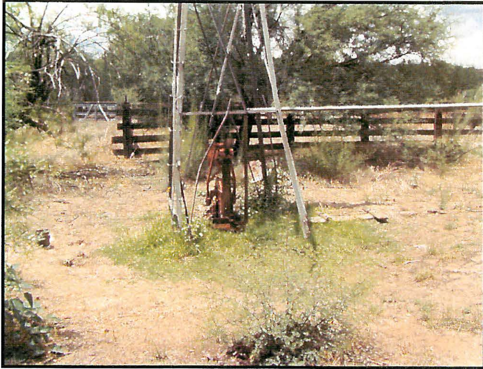
Windmill well upgrade. N332°W. Install 1 ½ HP submersible pump and motor.
