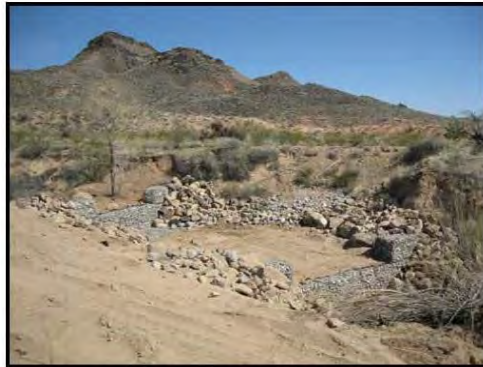
Site 2 and Site 2A construction sequence completion March 2012.
