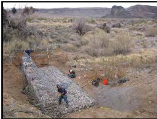
Site 3 construction sequence March 2012.
