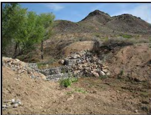
Site 1 post-construction upstream view April 2012.
