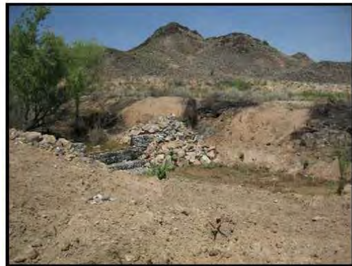
Site 1 post-construction upstream view April 2012.
