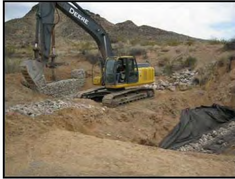
Site 2 and Site 2A construction sequence March 2012.
