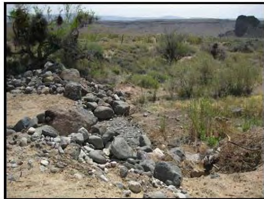
Site 3 construction sequence completion March 2012.
