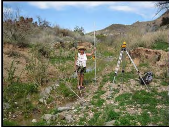
Site 3 pre-construction upstream view March 2011.
