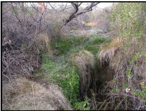
Site 1 pre-construction upstream view March 2011.
