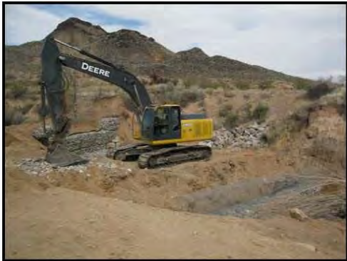
Site 2 and Site 2A construction sequence March 2012.
