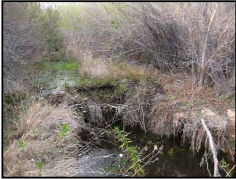
Site 2 pre-construction upstream view March 2011.
