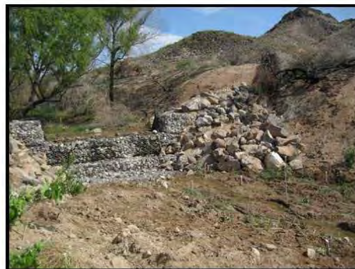
Site 1 post-construction upstream view April 2012.
