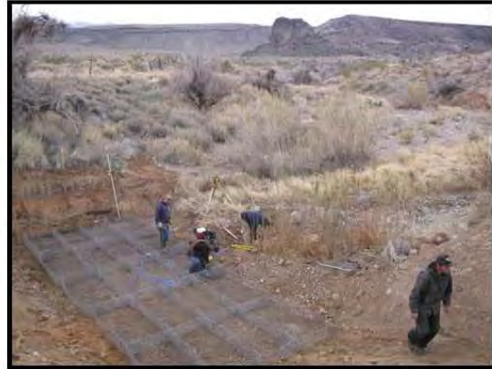
Site 3 construction sequence March 2012.
