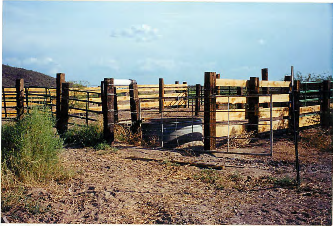
LOWER TNC CORRALS. PROPOSED SITE FOR WATER STORAGE, STOCK DRINKERS, AND CORRAL RE-DESIGN. (SOUTHWEST ORIENTATION)
