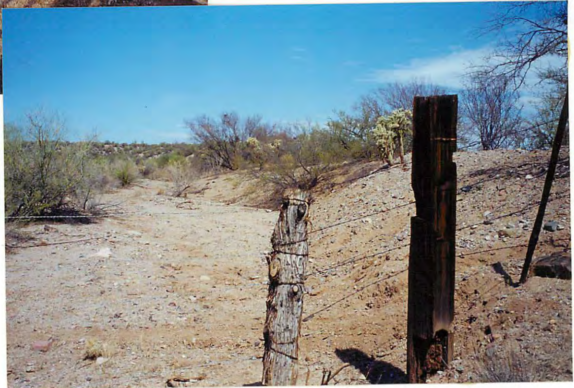
DOUBLE CHECK PERIMETER FENCE. ~ SITE OF LOWER TIE-IN OF DODSON CROSS-FENCE (WEST ORIENTATION)
