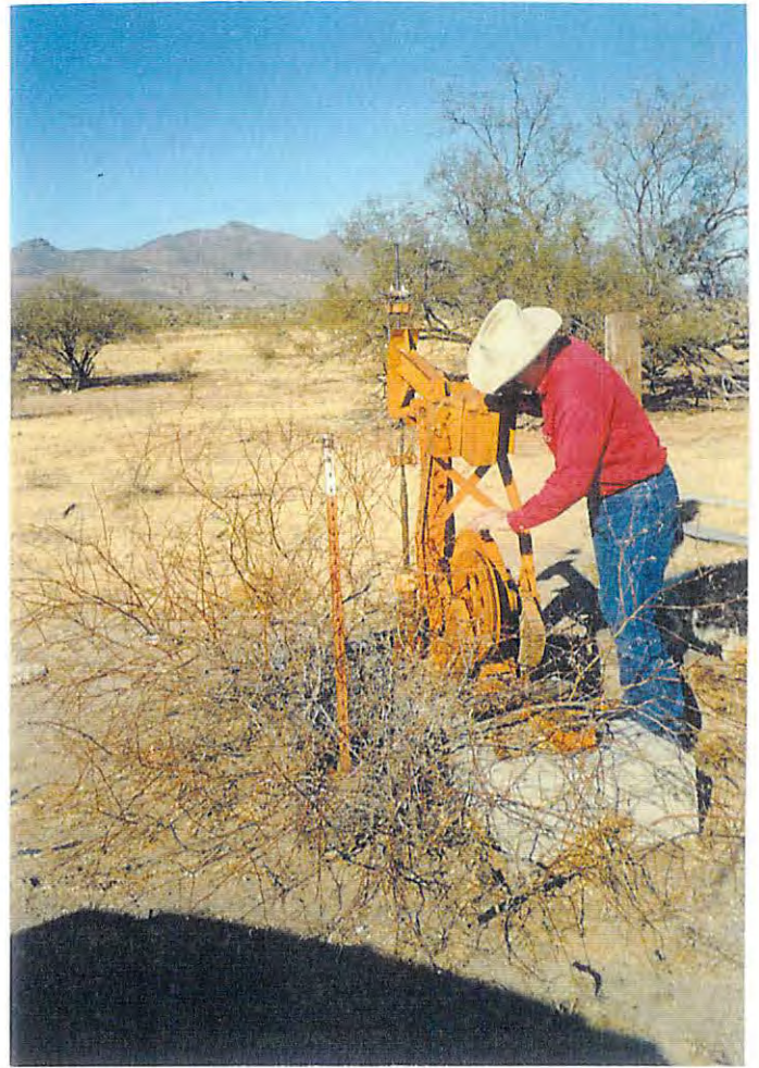
Buck Tank well with existing pump jack/ looking northwest
