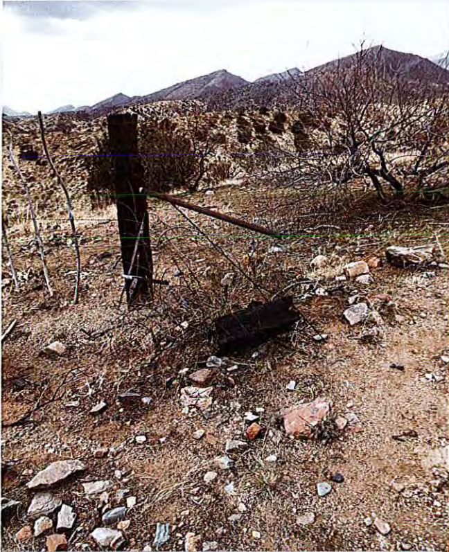
Partially burned fences have become a wildlife/livestock hazard. Heat causes the wire to become brittle, wood posts and stays are burned causing the wire to sag. Removal and rebuild are required to restore range health and barrier requirements.
