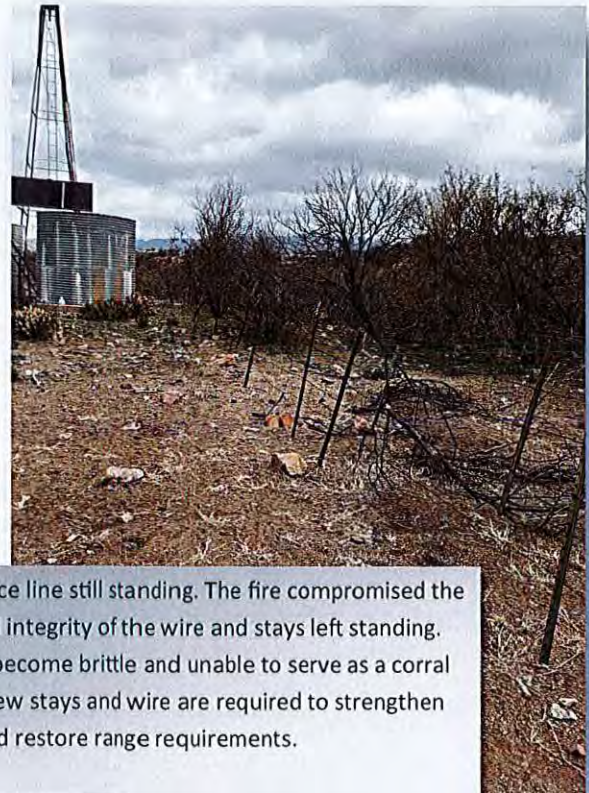
Example of sagging fence line that has become a wildlife/livestock hazard. Partially burned stays remain.
