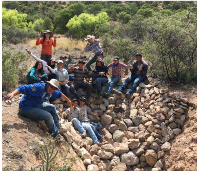
Figure 3. BECY interns proud of their loose rock structure, healing an 8-foot headcut.
