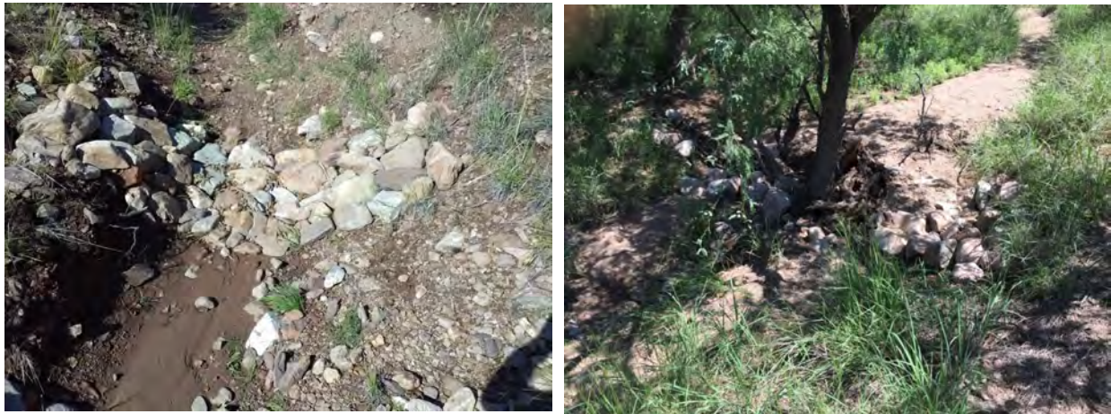
Figure 2. (Left) With flow direction from bottom of image to top, fine sediment is retained along with organic material that builds soil, while the passive structures allow water to continue flowing downstream. Structures become part of the system's ecological infrastructure and prevent further down-cutting and hydrologic draw-down that de-waters entire watersheds if left unabated. (Right) Approximately 18 inches of sediment and organic material (upper right) captured behind a low structure built into an existing tree and channel banks that were compromised.
