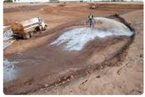
meet the most stringent wastewater standards utilizing on-site soil. With this method, the product is simply sprayed onto a properly prepared subgrade, and then allowed to dry. Once it is dry, a six-inch compacted soil cover is placed over the liner to protect it during the filling process.
